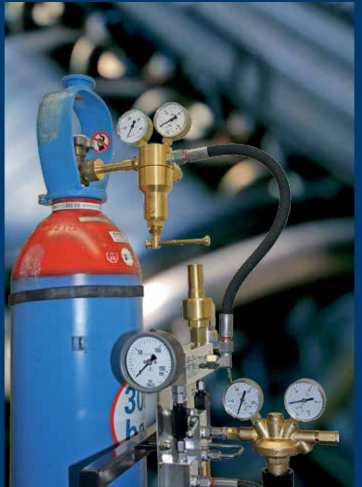
Leak test of the air-conditioning system with the KLDS 01.
