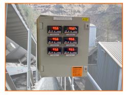
in the bitumen control room provides voltage level outputs for the site's upgraded PLC currently being installed. Using the standard external aerials, the radio system has a minimum working range of 200 metres, increasing to 500 metres with good line of sight. This can be upgraded using higher power aerials.
