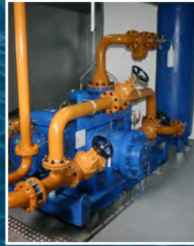
Metering system for diesel measurement
